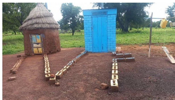
Household latrines constructed with Interlocking blocks in Takuka
